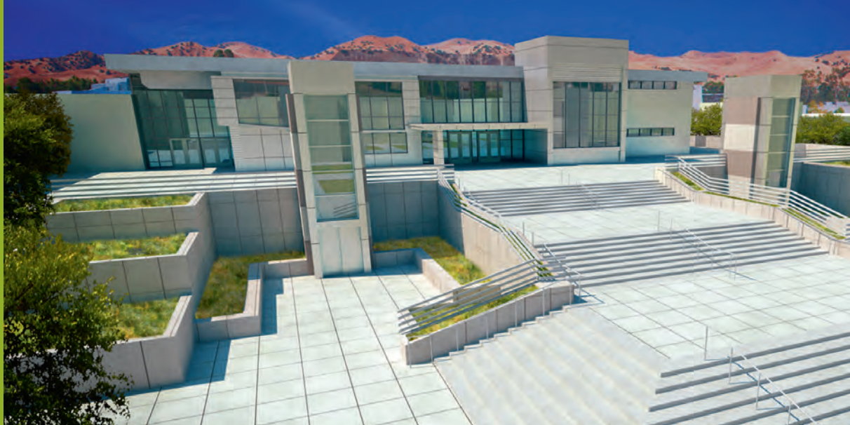
Top: Groundbreaking of the CCC College Center project, which will include a new Classroom building. Right: Culinary Arts on the upper floor and the Food Services Dining Room on the lower floor of DVC Commons' north wing. Bottom: LMC College Complex project. Project renderings by Steinberg Architects and tBP/Architecture.
