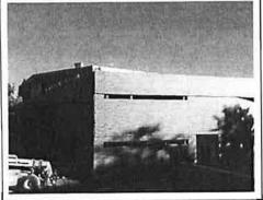
COMMENTS: Phases 1, 2, and 3 are complete. Phase 4 construction of the new Food Services and HRM building is proceeding on schedule. The exterior wall panels have been installed and roofing is approximately 40% complete. Installation of curtainwall and glazing is well underway, along with mechanical, electrical, and plumbing systems. Interior wall framing is nearly complete. The Project remains on schedule.
