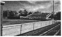
COMMENTS: Goodland Landscape Construction has finished all drainage, irrigation, grading, sod installation, and construction of the backstop walls, bleachers fencing, backstop netting, and dugouts. Substantial completion is expected mid December. The campus begins field maintenance on 12/23/2013. Bleacher ramp modification to take place in January. Fields are scheduled for campus use in January 2014.
