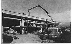
COMMENTS: Project is in progress. The following work activities have been completed: structural steel, steel fireproofing, concrete shear walls, roof membrane, mechanical curbs and piping supports, skylights, fire main lines, interior concrete slabs. The following work activities are in progress: exterior metal framing and insulation, rough ins for mechanical, plumbing, fire sprinklers and electrical.
