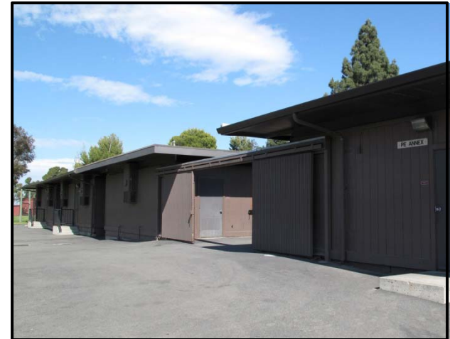
Existing Men's and Women's Locker Rooms
